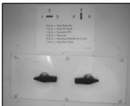
**Fig. A Water Valve Controls**
